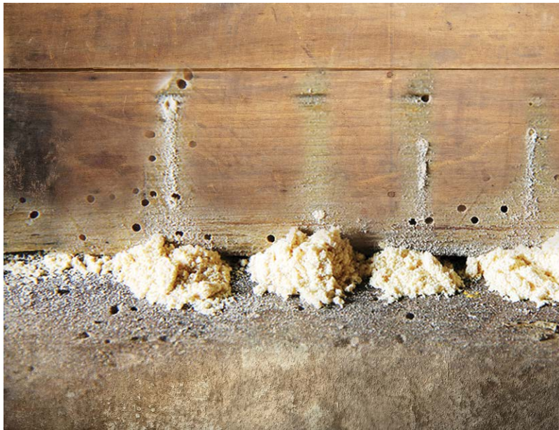
Fig. 7.5. Fine wood powder being pushed from the exit holes of powderpost beetles. (Courtesy of Dr P. Suresh.)
