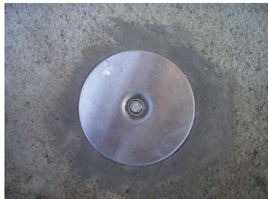
Fig. 11.13. An in-concrete station in place. (Author's photo.)
