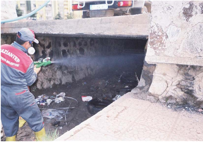
Fig. 4.10. Using handheld low-volume applicator to treat space in inaccessible areas. (Courtesy of Biosav.)
