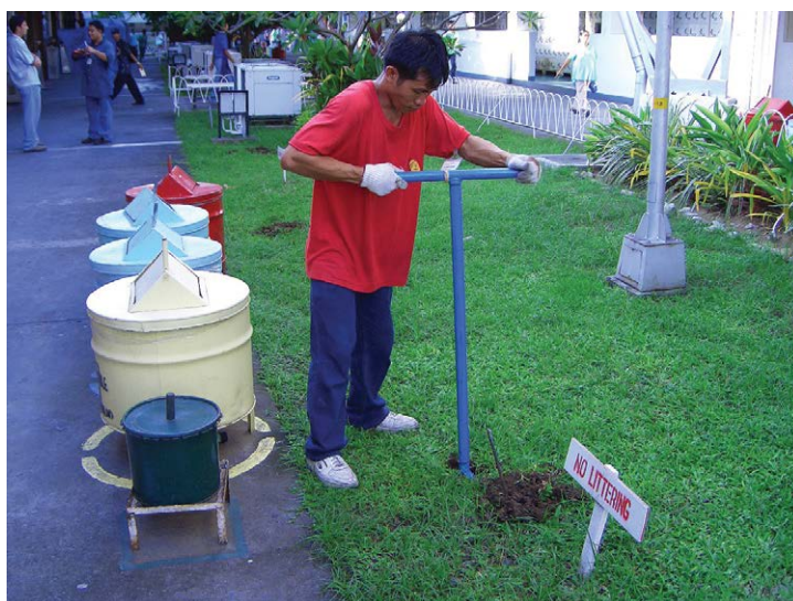
Fig. 11.8. Use of a handheld augur to make a hole for the in-ground station installation. (Author's photo.)
