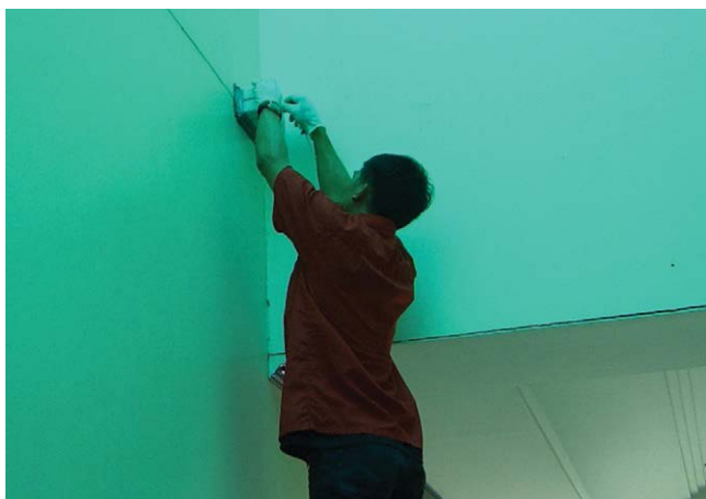
Fig. 6.24. Installing an above-ground baiting station on an active site. (Author's photo.)
