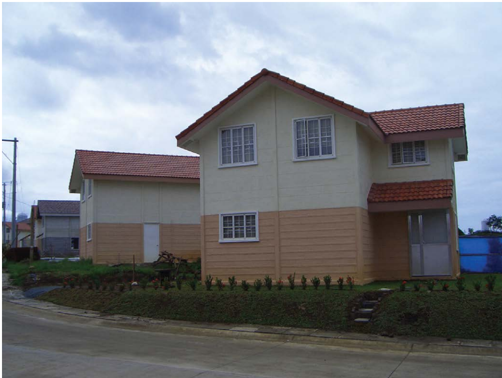
Fig. 6.23. Houses built in newly developed areas by land developers are highly susceptible to termite attack. (Author's photo.)
