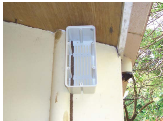
Fig. 6.28. Positioning an above-ground station over a mud tube correctly before baiting. (Author's photo.)
