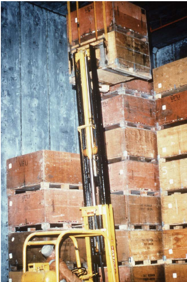
Fig. 8.1. The inside of a traditional controlled atmosphere store in England showing the internal walls covered with galvanized sheets to render them gas tight. Photograph courtesy of Dr R.O. Sharples.
