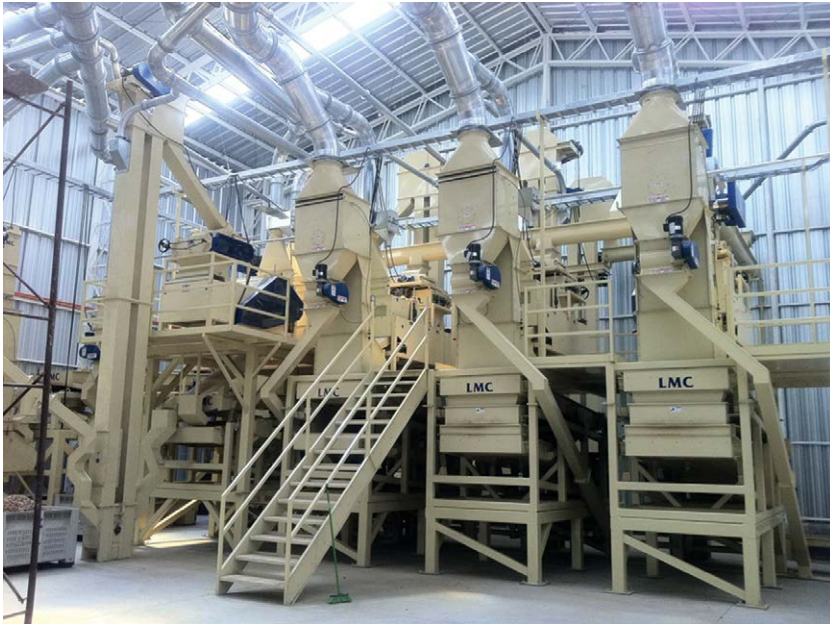
Fig. 20.2. Almond processing plant. Cracking. (With kind permission from SIRVENT ALMENDRAS S.A. – http://www.sirventalmendras.com .)
