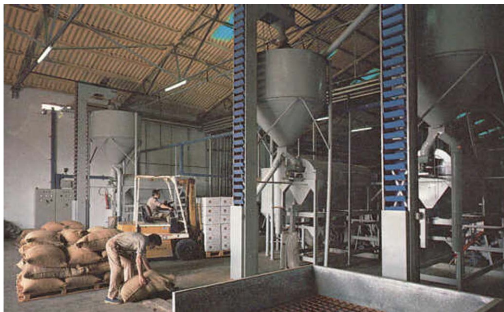
Fig. 20.1. Almond reception plant. (With kind permission from SIRVENT ALMENDRAS S.A. – http://www.sirventalmendras.com .)
