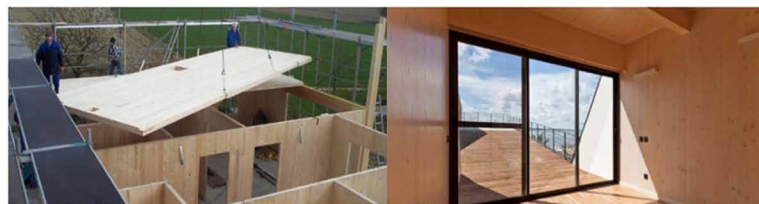
Figure 2. Construction with CLT panels (Source: https://www.jular.pt/produtos/placas-e-paineis/paineis-clt ).
