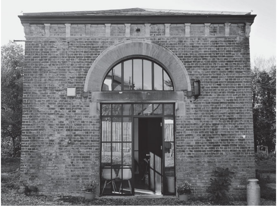
4.2: Uchronia Workshop 1 , Pumping Station in Cheshunt, 2014 Photograph: students (Group Two)
