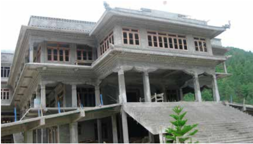
Figure 16b Ongoing construction of Thupsung Dhargyeling Monastery 2013
