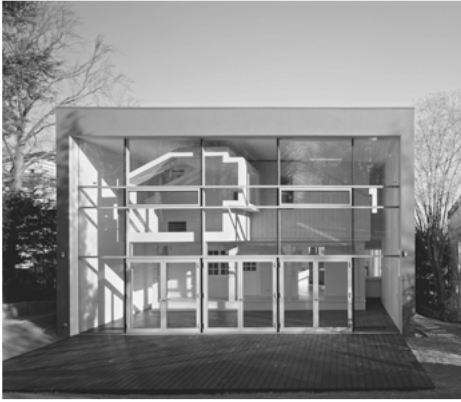
Fig. 42: An existing house is rebuilt using a second house: the concept of a house within a house.
