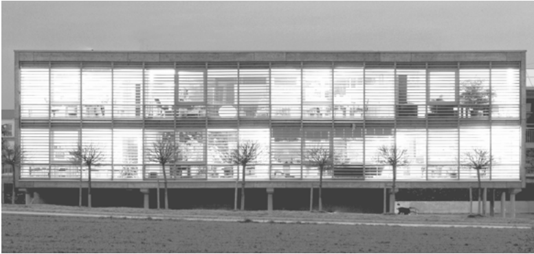
Fig. 34: A glazed facade as a transition between interior and exterior
