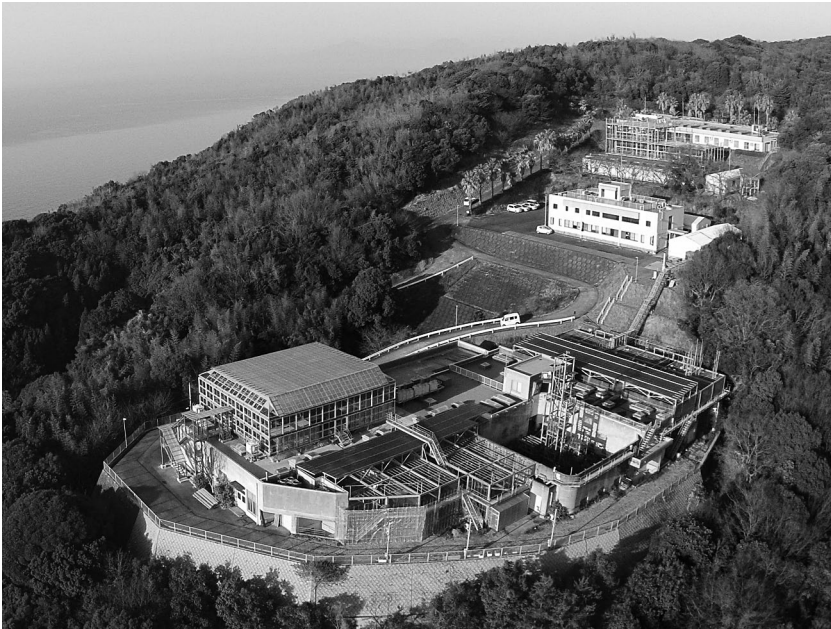
FIGURE 9.3. Aerial view of Kumamoto Sanctuary, Japan.
