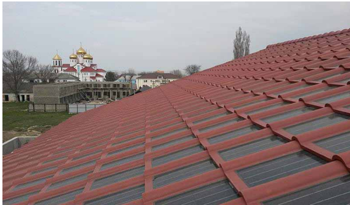
Figure 7. “Solar House” in Anapa with a living area of 150 m 2 with a roof of a solar tile with an electric power of 2 kW
