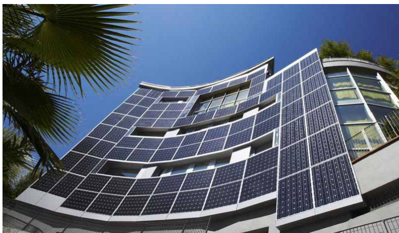
Figure 12. The exterior of the outer wall of the building with solar panels (USA, California)
