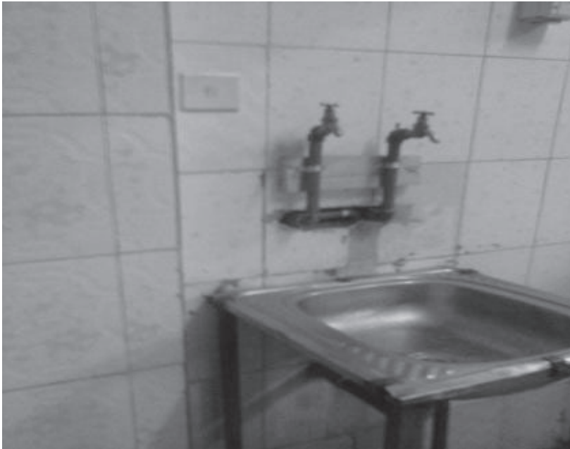
Figure 7-1: Separate hand washing sink for food handlers without soap and hand drier
