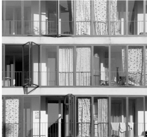
Fig. 3: Local visits can show whether users have accepted the intended use of a building.
