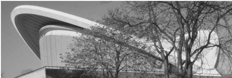
Fig. 70: A reinforced concrete hyperbolic paraboloid
