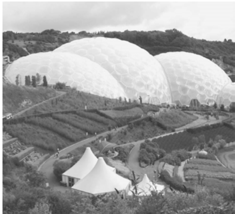
Fig. 53: The Eden Project in Cornwall
