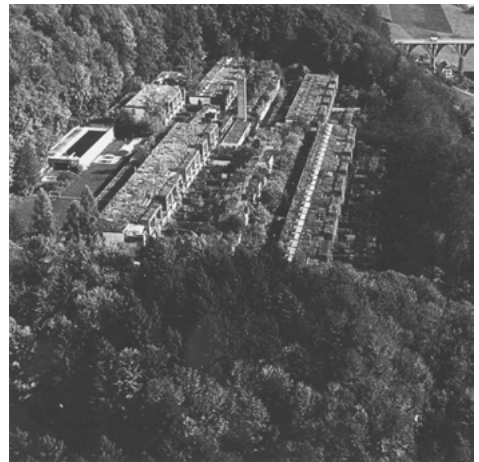
Fig. 83: The “island” leitmotif for the design of a housing estate in the forest
