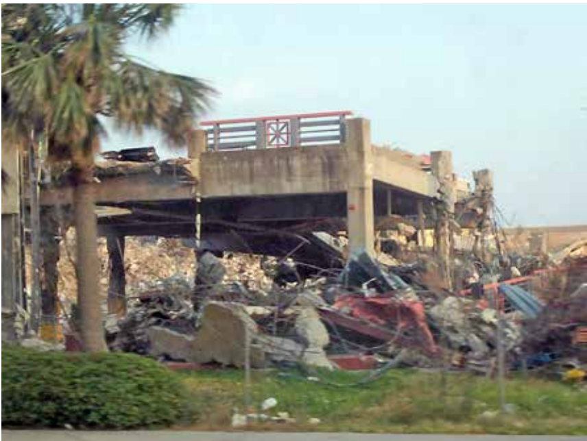
Figure 3.4 Grand Casino Damage. Source: Created by Jennifer Trivedi.
