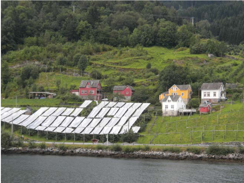
Fig. 9.7. These structures for rain covers, located in Norway, are made out of wood, but can be susceptible to damage by high winds (courtesy of L.E. Long).
