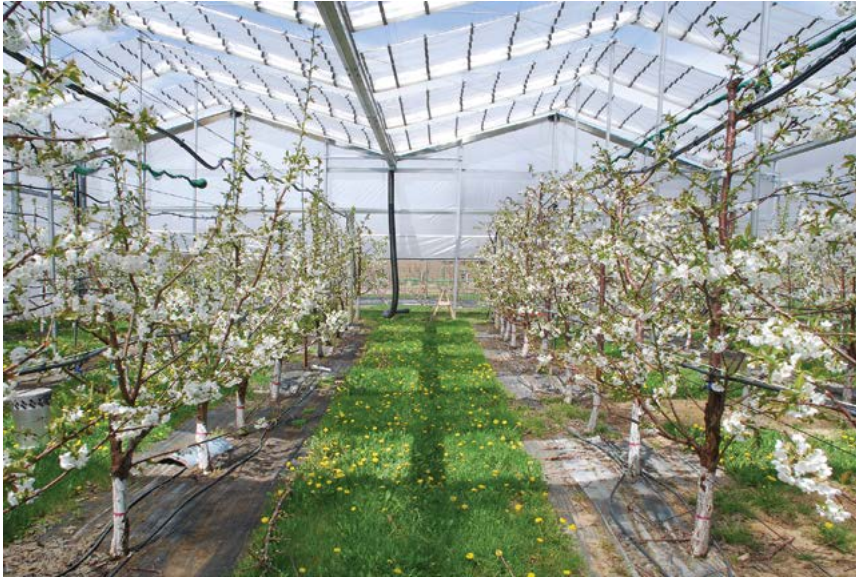
Fig. 5.18. Cravo brand greenhouse retractable roof partially open to balance heat retention and facilitate honeybee navigation for pollination (courtesy of G.A. Lang).
