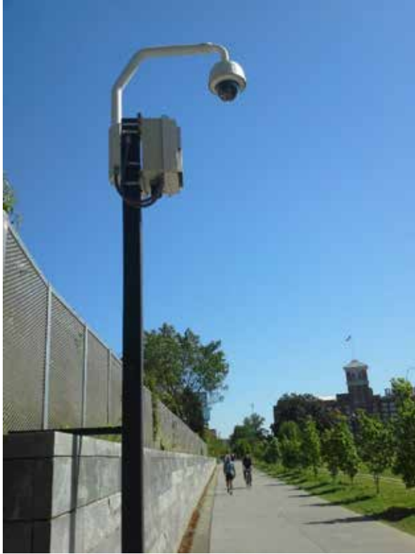
Figure 4.2 Security Camera Under Dome Cover, Beltline Park, Atlanta, USA. Source: Photo taken by author.
