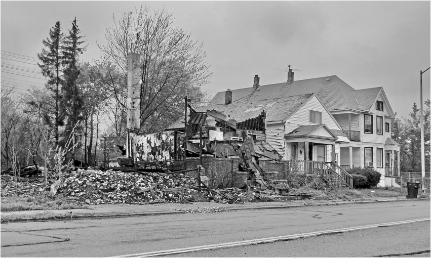
Photo 1. A deteriorated, fire-damaged house in Detroit; the house next door has melted siding from the heat of the fire. Photo credit Michael Brown
