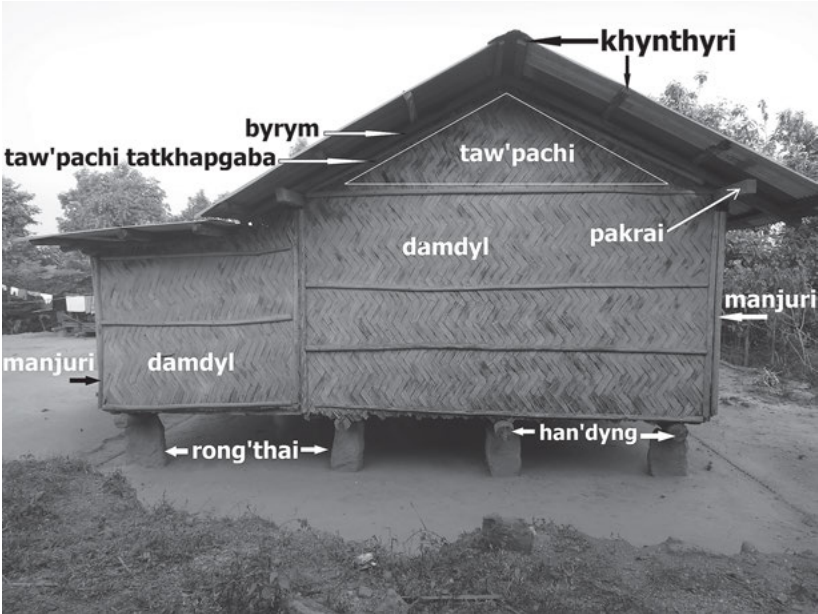
Photo 10: Parts of the house (2), side of the house (adapted from van Breugel 2014: 635).
