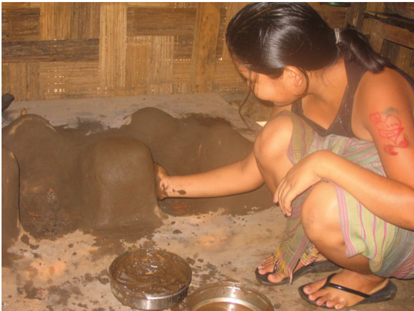
Photo 17: Radia D. Sira chula ryphigaba 'plastering the cooking place'.
