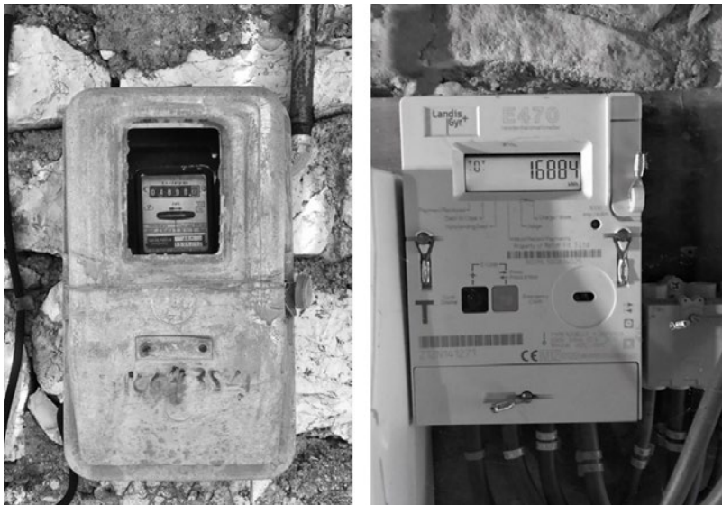
Figure 6.3. From the temporally imprecise and infrequent data making rhythms of manually read meters, to the high precision and high resolution rhythms of smart meters.
