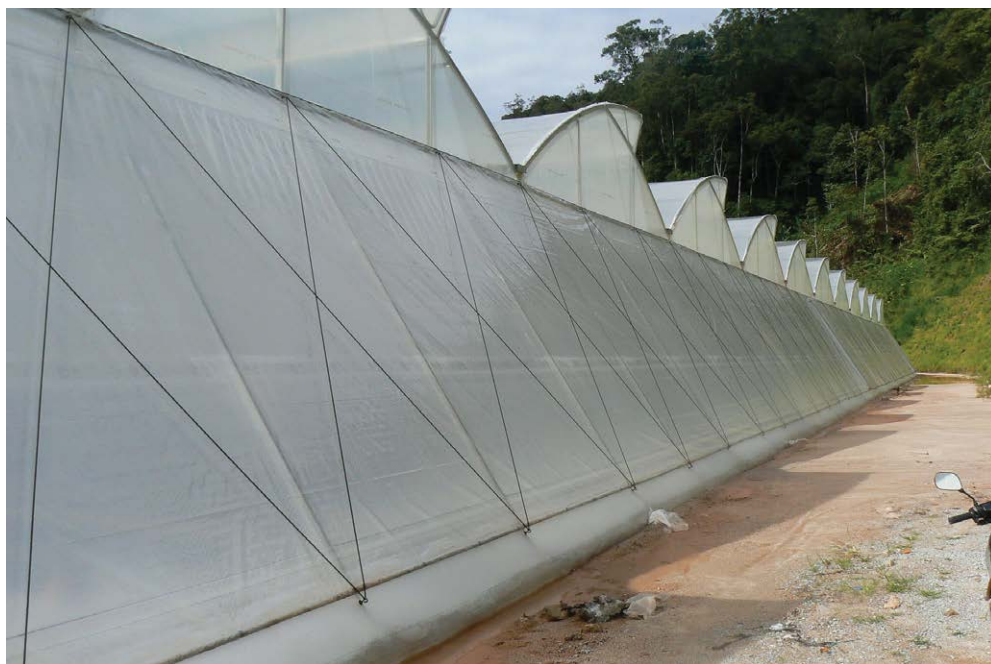
Fig. 2.2. Greenhouse design which consists of a number of connected arches.
