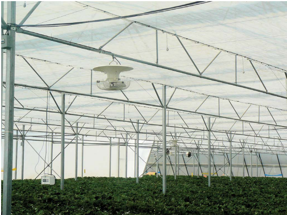
Fig. 3.5. Vertical air-movement fans assist air movement and humidity control.
