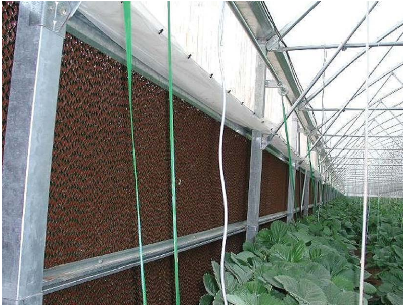
Fig. 3.2. Fan and pad evaporative cooling wall.
