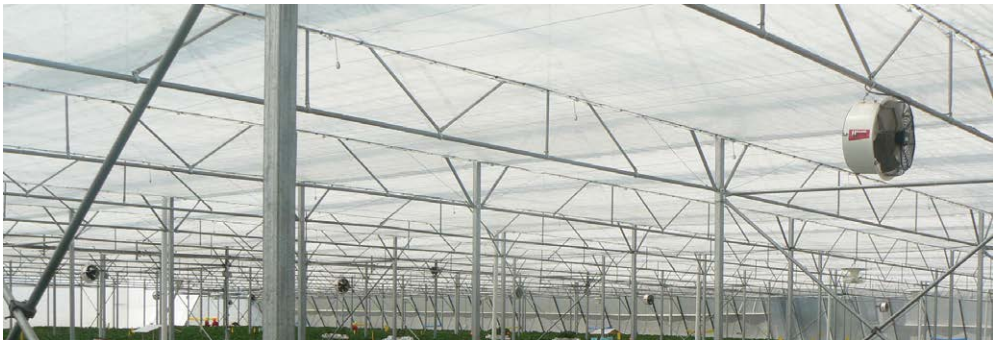
Fig. 3.4. HAF fans positioned to circulate air within the greenhouse.
