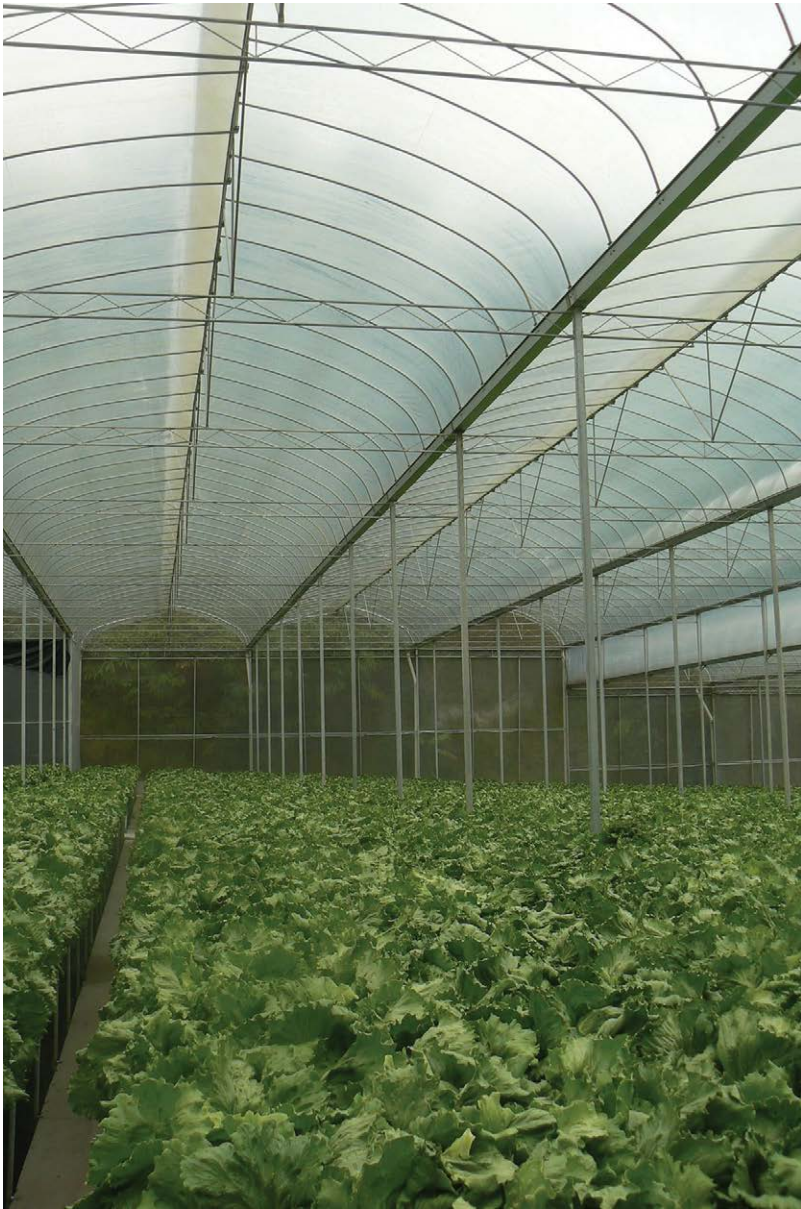
Fig. 2.6. High tunnels are a form of low-cost greenhouse using natural or passive ventilation.
