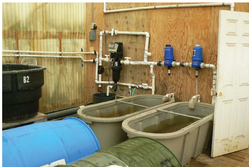
Fig. 6.12. Nutrient tanks and Dosatron injectors.
