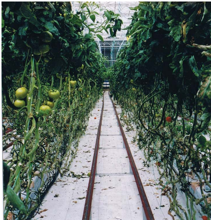
Fig. 3.1. Hot water heating pipes.
