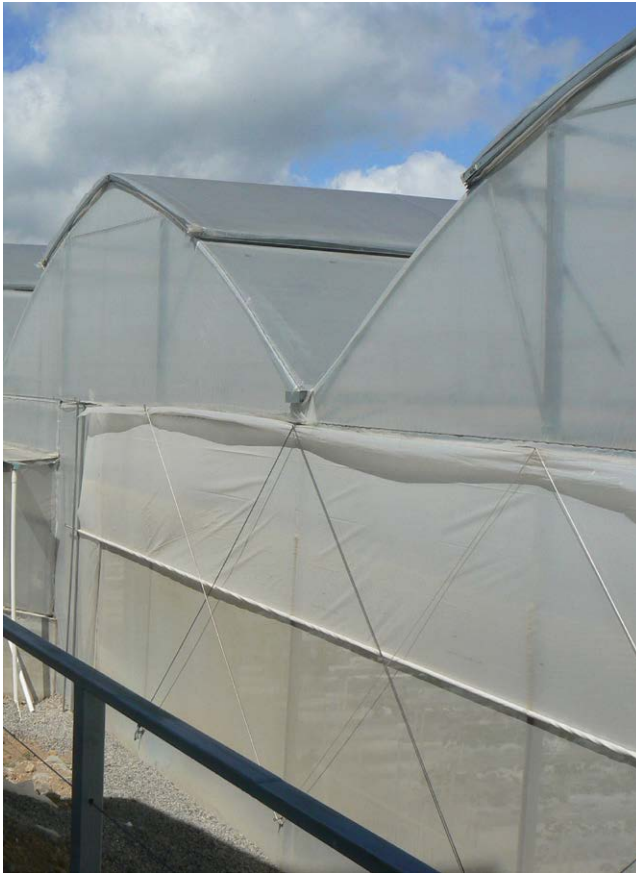
Fig. 3.3. Greenhouse top and side vents.
