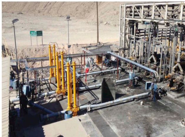
Figure 15. Tailings pumping plant at Coemin with VPD.
