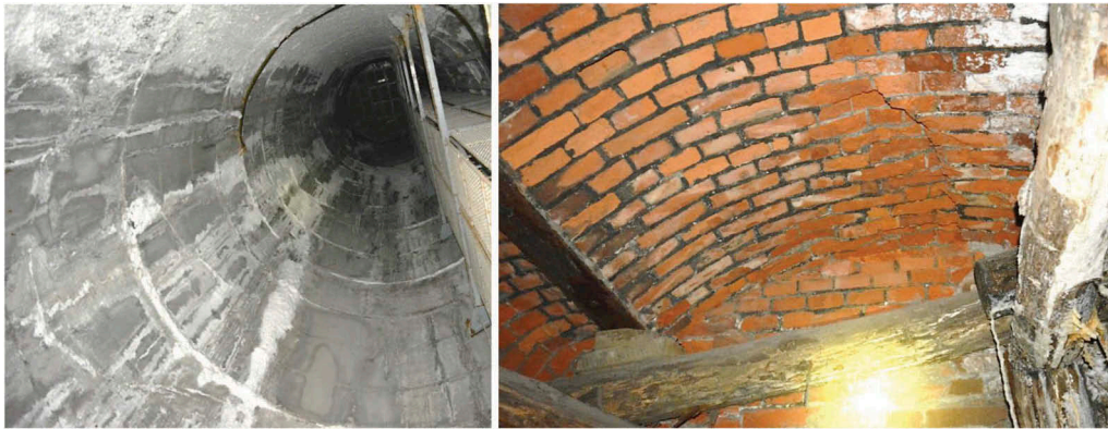
Figure 6. Damage to the shaft lining and shaft bottom supports occurring in the vicinity of the level IV.
