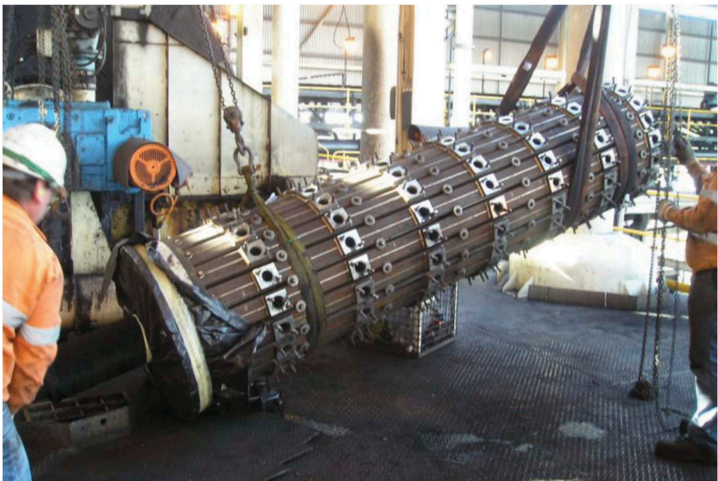
Figure 6. Lifting of new filter barrel.
