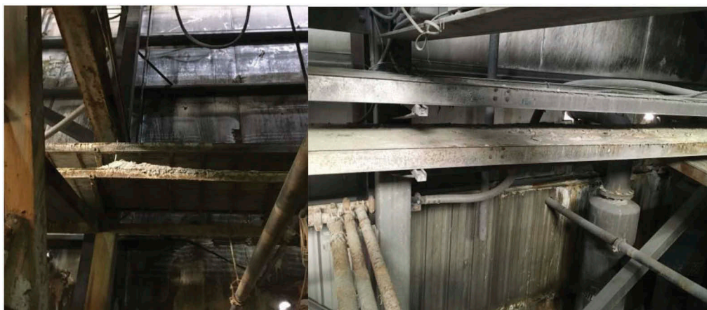
Figure 10. Cable tray's full and corroded/full of tailings.
