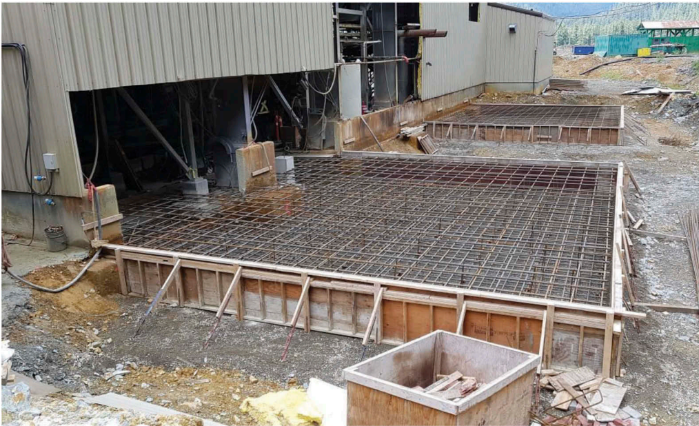
Figure 8. Silo and filter feed tank raft footings.
