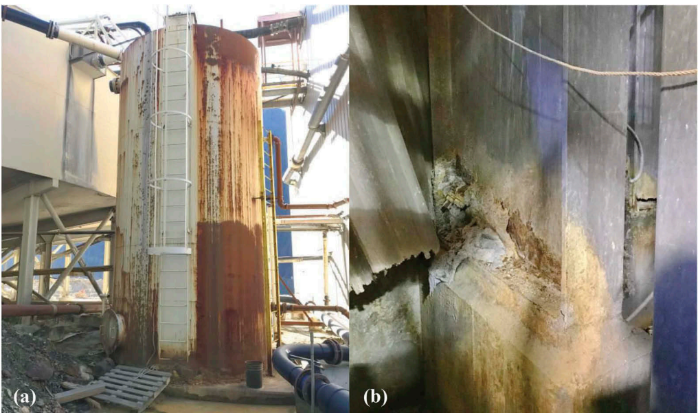
Figure 7. Examples of existing equipment corroded from contact with tailings (a) Process water tank and (b) Building column.
