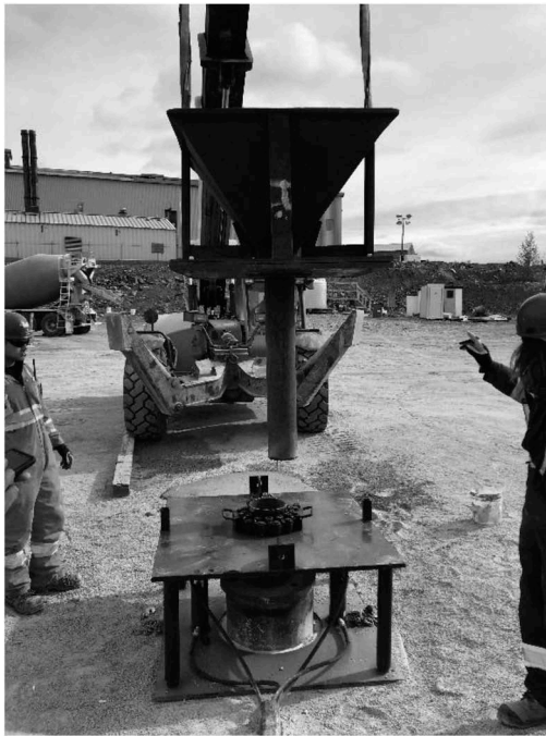
Figure 6. Hydraulic jacks for raising the tremie pipes.
