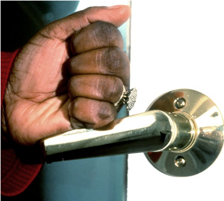
Figure 3.4. Fist pushing down on a lever door handle demonstrating that it does not require the strong grip needed by a round doorknob.
