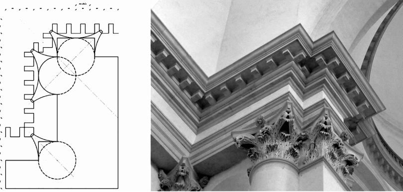
FIGURE 10. In Il Redentore, pilasters comply to the module, while the modillions in the cornice create an odd condition at the inside corner.
