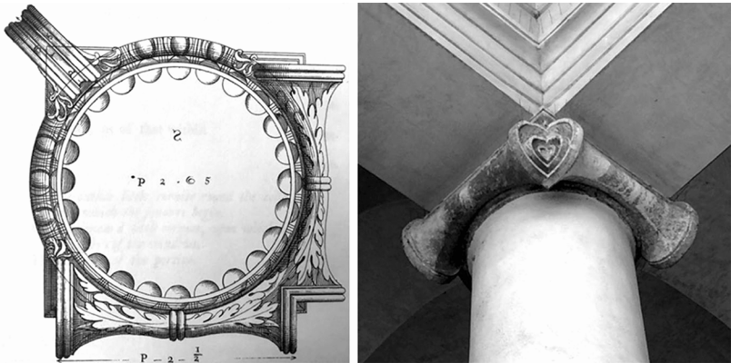
FIGURE 3. Turning the corner with an Ionic column presented architects with a difficult formal challenge. At the outside corner, the volute was adjusted on a 45^\circ angle to make the turn, while on the inside corner, the two volutes merely collided, as can be seen in the Palazzo Barbarano of Palladio. [Drawing by Palladio, Book IV.]
