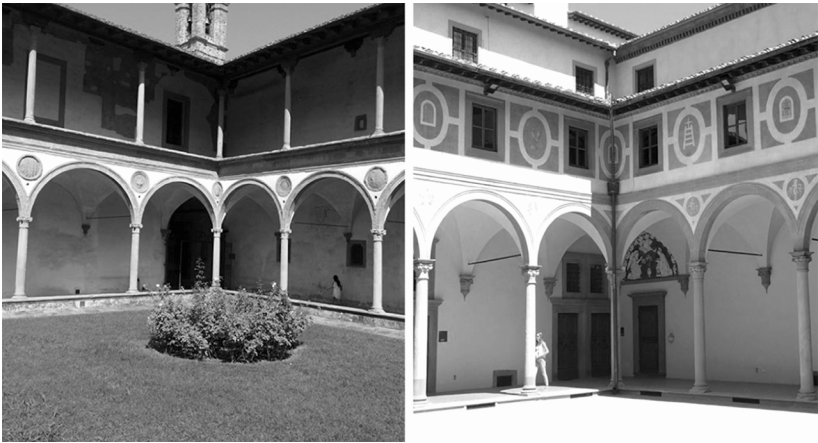
FIGURE 2. Two fifteenth-century Florentine interior courtyards, Santa Croce (left) and Ospedale degli Innocenti (right), show that a rigorous module of columns leads to compromised spandrel conditions at the inside corner.
