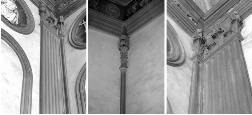
FIGURE 12. Pilaster fragments occur at the typical interior corners of the Pazzi Chapel.
