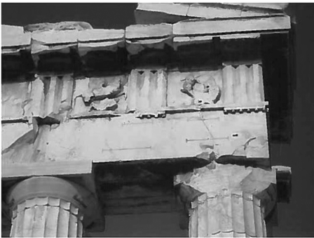
FIGURE 7. The rules of the Greek Doric order required that the corner of the frieze be turned by a full triglyph. This meant that either the regular spacing of the columns was maintained at the sacrifice of the last metope (drawing above), or that the column spacing at the corner be reduced to permit a consistent frieze (drawing below). (Drawing from Durm 1892. This image is from Tzonis and Lefaivre 1986.)
