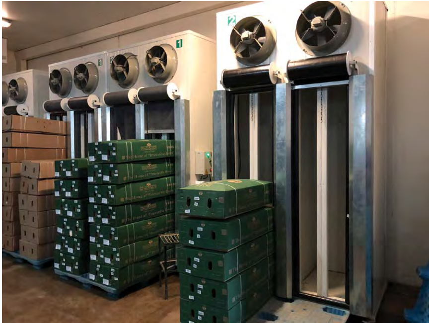
Fig. 8.15. Forced-air cooling allows rapid removal of heat from within boxes of flowers. (Photo: J. Faust.)
