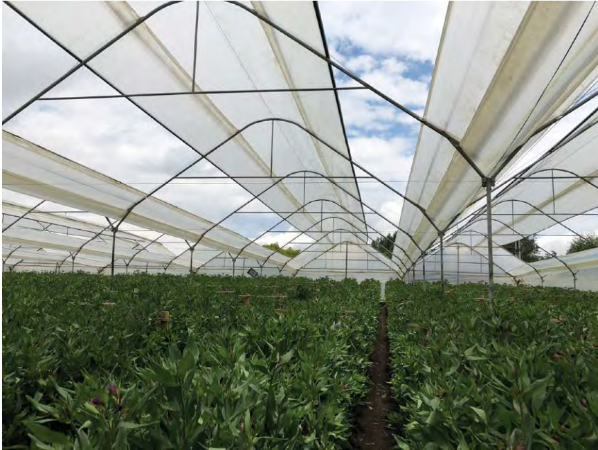
Fig. 2.1. A retractable roof greenhouse is used on an alstroemeria crop to allow for higher light levels (DLI) while rainfall or excessive winds are not a concern. (Photo: J. Faust.)
