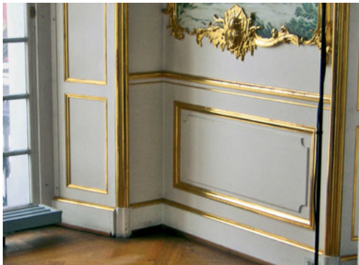
Fig. 8-9 Wood cladding in a historical building: details of the construction concealed behind the cladding are undistinguishable.
