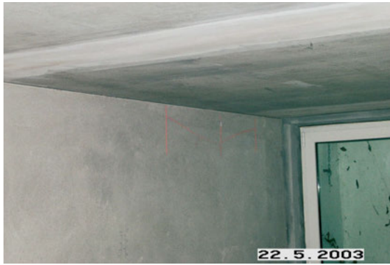
Fig. 7-82 Joint of the basement concrete ceiling and the masonry partition wall, elevated surface temperature near the window: a subsequent uncovering of the construction part revealed missing thermal insulation and clumps of concrete at the height of the ceiling.
