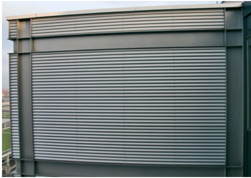
Fig. 7-70 View onto the rear-ventilated facade construction made of corrugated sheets. The angle of perspective changes continuously between 0° and 90° from one corrugation to the next (also see Fig. 2-14).
