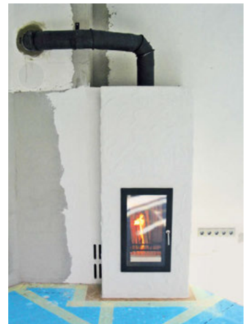
Fig. 7-59 Arrangement of the coring to transfer the weight of the fireplace to the ground slab ( left ); first heating of the installed fireplace ( right ).
