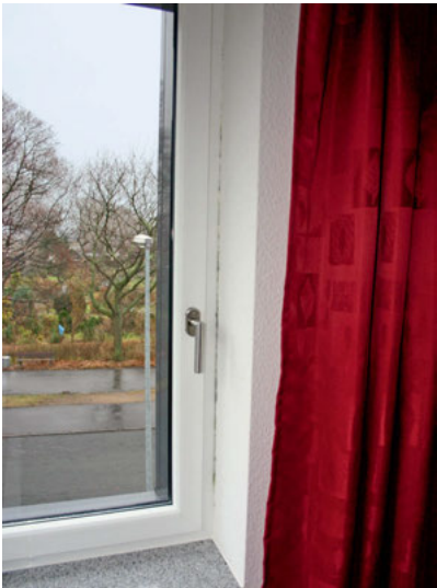
Fig. 7-86 Overview of the apartment building with brick facing: The renter complained about mold formation at the transition between the window frame and the reveal.
