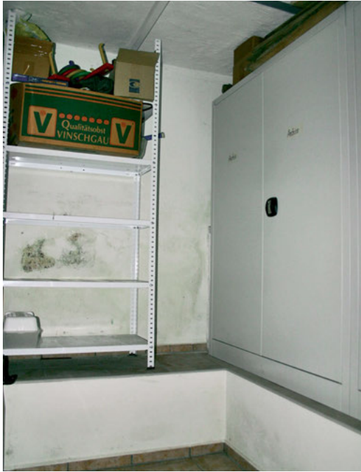
Fig. 7-44 Stains on the plaster show the moisture influence.
