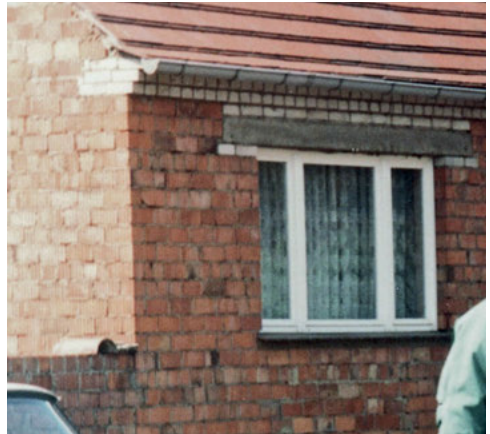
Fig. 7-6 Masonry construction with uninsulated lintel (reinforced concrete); (right) photograph taken during the construction process (approx. 1986) showing the position of the window lintel made of concrete.
