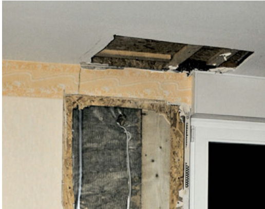
Fig. 7-34 Uncovered examination area between the wall and ceiling and respective thermograms before and during the application of low pressure (about 50 Pa).
