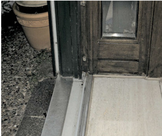
Fig. 6-12 Thermally isolated threshold of a terrace door.
