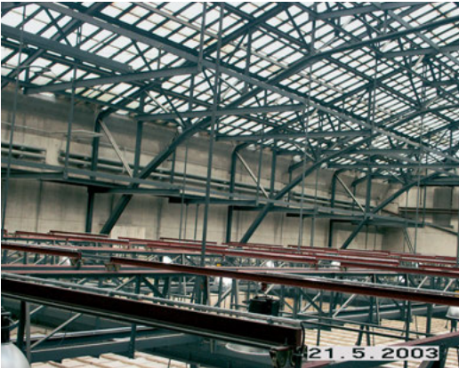
Fig. 7-68 Tied arch construction of an open-sided floor.
