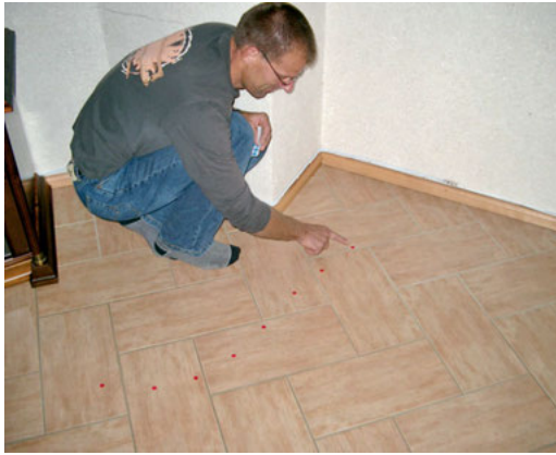
Fig. 7-57 Pipe run shown under the parquet floor ( right ). The location of the heating pipes is documented with the aid of glue dots on the floor ( left ).
