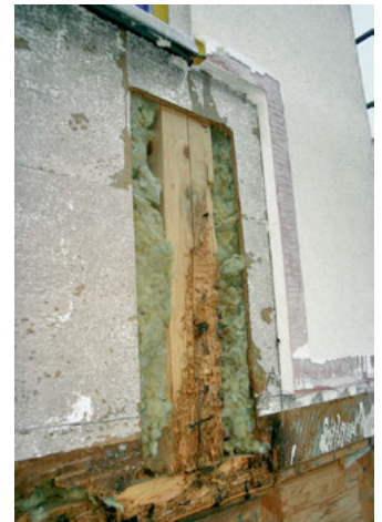
Fig. 7-26 Residence building with exposed examination point in the region of the ceiling slab. The external construction is removed all the way to the thermal insulation.
