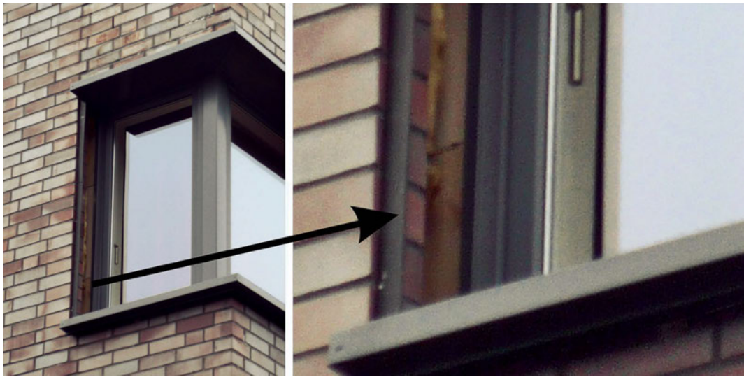
Fig. 7-88 Uncovered exterior cover plate: (right) close-up of the detail, showing that the thermal insulation had not been fit properly to the reveal.
