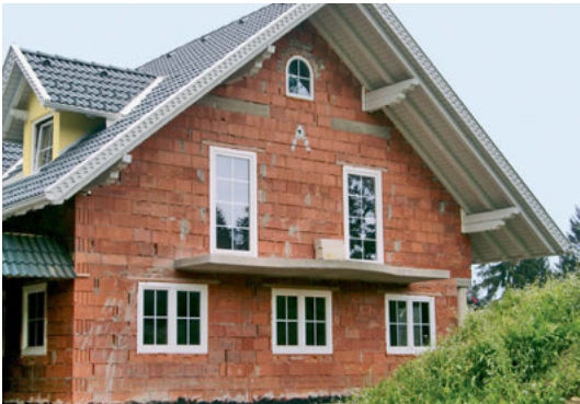
Fig. 6-5 Typical example of a potentially critical thermal bridge: cantilevered reinforced concrete slab of a balcony, in this case without correct thermal isolation.
