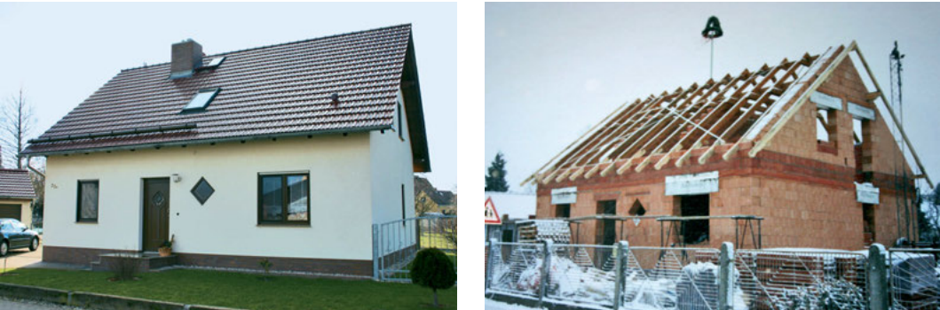
Fig. 7-13 Residential building at the time of the thermography measurement ( left ) and at the time of construction ( right ): above the windows, insulated roller blind boxes and the circular ring beams (U-shaped shells with reinforced concrete, see Fig. 7-20) are located.
