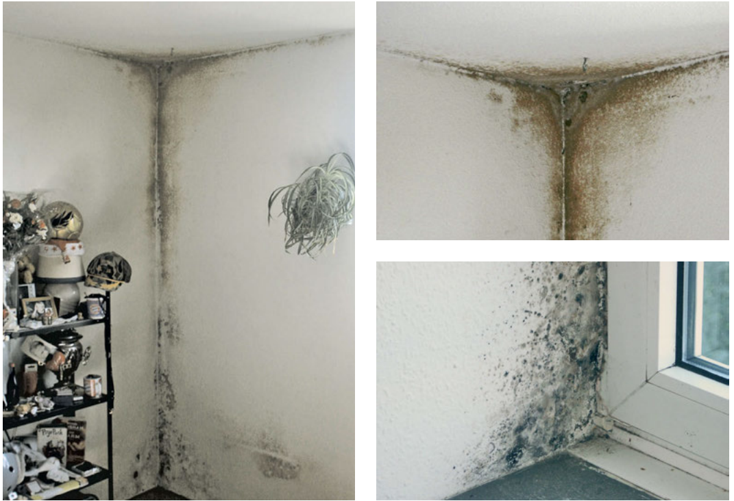
Fig. 6-15 Extreme mold formation on the inside corner between exterior walls and the ceiling and along the window soffit.
