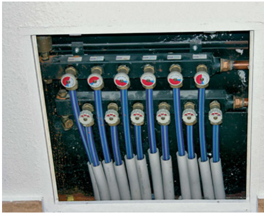
Fig. 7-56 An underfloor heating distributor; one valve of the pipes (second from left) is unopened.
