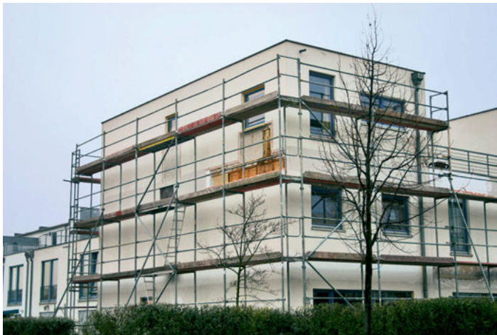
Fig. 7-26 Residence building with exposed examination point in the region of the ceiling slab. The external construction is removed all the way to the thermal insulation.
