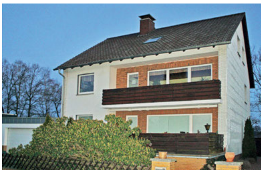
Fig. 5-15 Exterior perspective of the building, measuring of the surface temperature in the exterior ceiling corner (left side of the balcony on the upper floor) by means of a contact thermometer; displayed measuring value: \theta_{se} = 11.1^\circ\text{C} .
