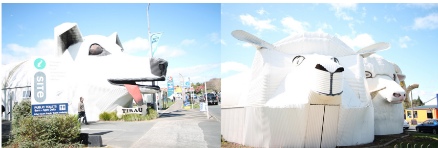
Figure 3.2 "Big Dog" Toilet Block and Information Centre and "Big Sheep" Wool Gallery, Tirau, New Zealand. Source: Photo Credit Diane Johnson.
