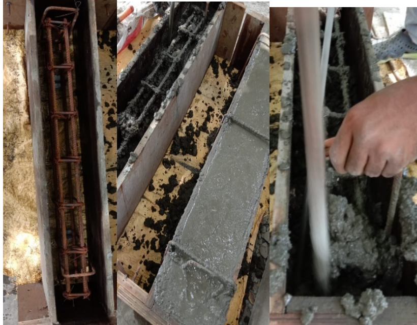
Figure 4(b). Beam reinforcement and casting
