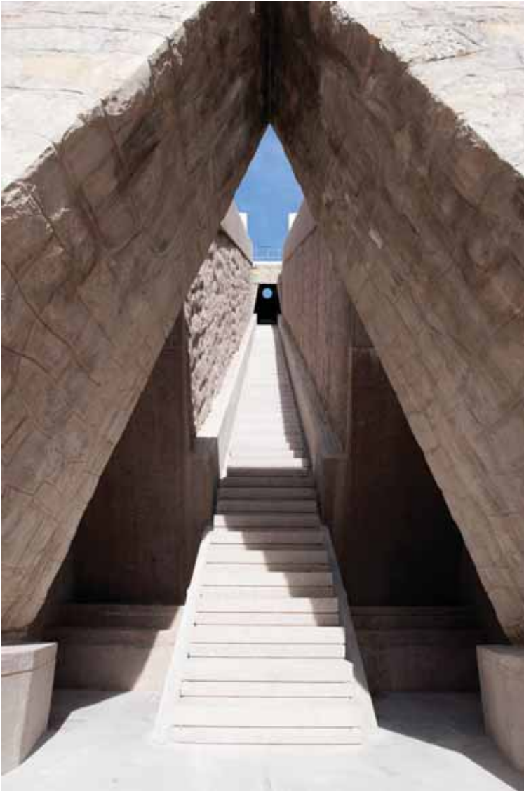
Fig. 5-3. Star Axis, Star Tunnel. The stairs in the Star Tunnel are exactly parallel to the axis of the earth. Credit: © 2021 Charles Ross / Artists Rights Society (ARS), New York
