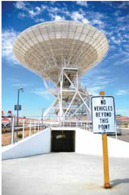
Fig. 5-2. The DSS-13 RARG / VENUS antennae at NASA's Deep Space Network in Goldstone California.
