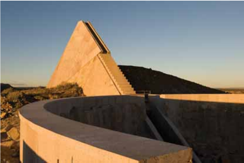
Fig. 5-5. Star Axis, Solar Pyramid Spine. The stairs on the spine of the Solar Pyramid are exactly parallel to the axis of the earth. The Solar Pyramid is actually a tetrahedron. The face of the Solar Pyramid is the angle of the sun at summer solstice and the back of the tetrahedron is the angle of the sun at winter solstice. Credit: © 2021 Charles Ross / Artists Rights Society (ARS), New York
