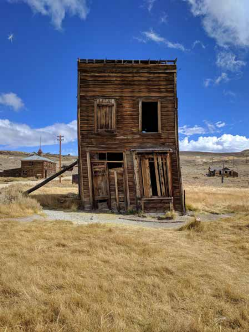
Figure 4.2. Arrested Decay at Bodie. Photograph by Author
