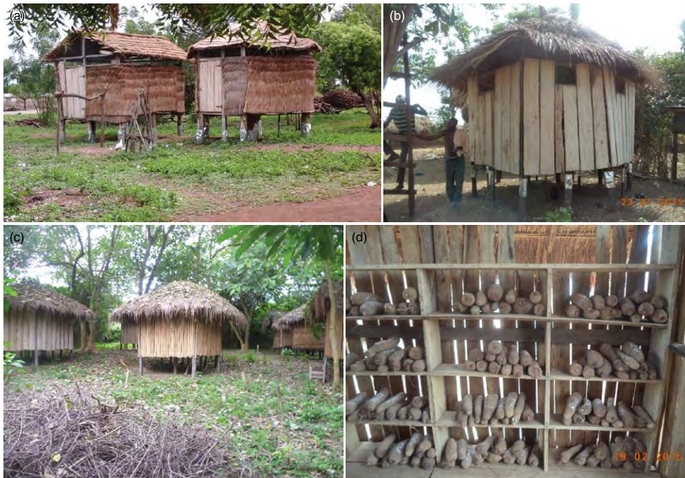
Fig. 5.2. Yam storage barns constructed with locally sourced materials: (a) Zanna mat covering; (b) wooden slabs from sawmill cut-offs for structure walls; (c) bamboo sticks for structure walls; and (d) storage shelves made from wood from the Kapok tree ( Ceiba pentandra ).
