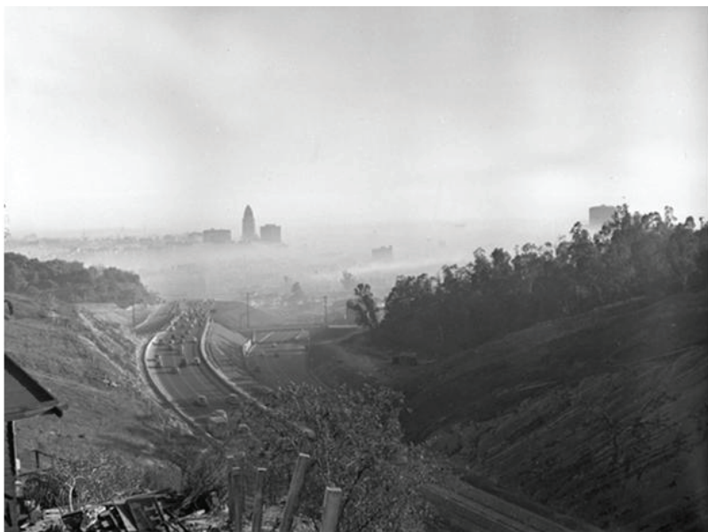
Fig. 1.2. A photo from above of Hollywood on 26 July 1943, looking eastward towards downtown Los Angeles. At that time, the largest building downtown was the city hall at 32 stories. The road shown is the beginnings of the Hollywood Freeway (now Interstate 10). If the photo were in color, the layer of smog would be brown. Photo from WIRED, Source: http://www.wired.com/thisdayintech/2010/07/07261a-first-big-smog/ , non-copyrighted
