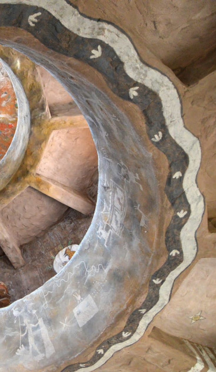
FIG. 5.7. Looking up at the Watchtower ceiling. Photograph by Margaret Randall.
