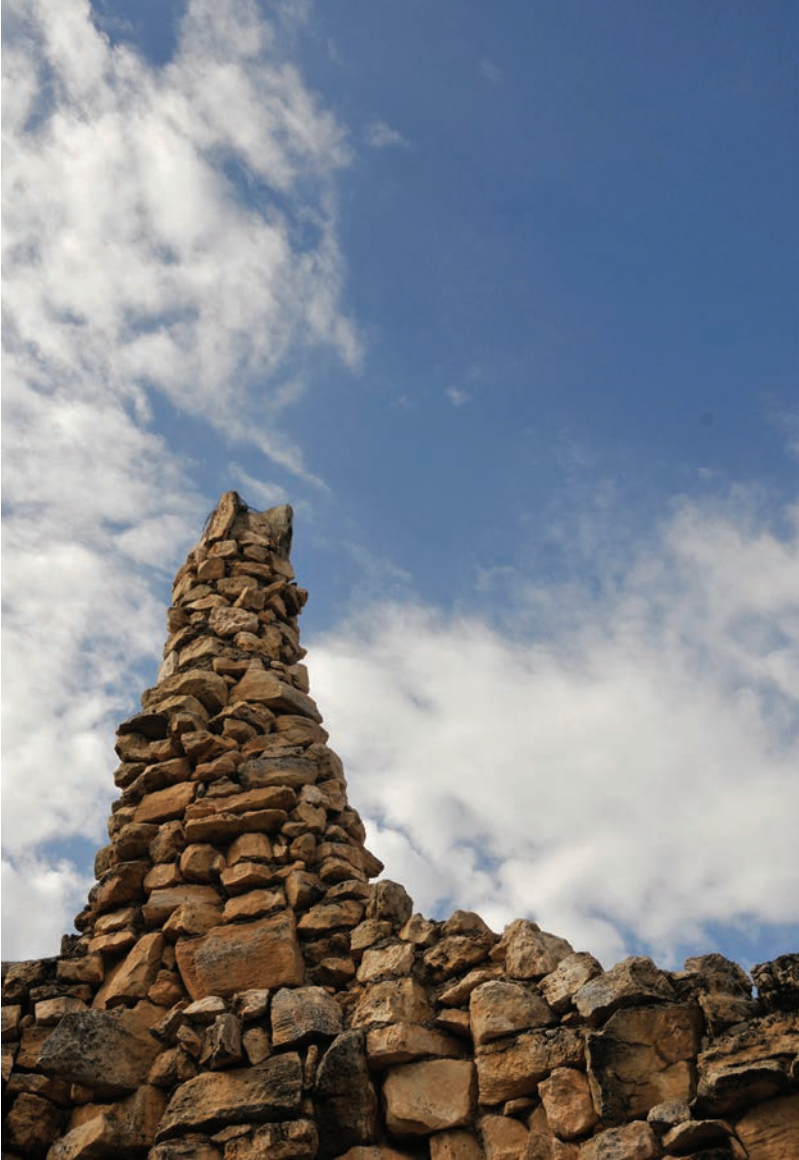
FIG. 5.1. Hermit's Rest chimney, Grand Canyon. Photograph by Margaret Randall.
