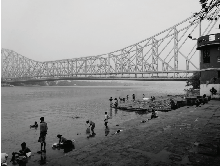
Howrah Bridge, Kolkata
