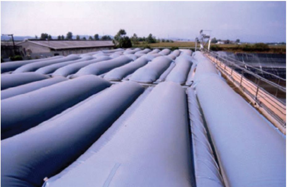
Figure 12.20: Biogas collection system from lagoons [127].
