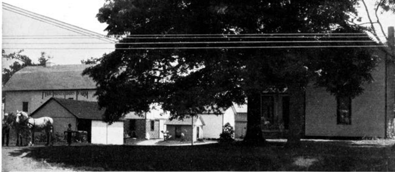
The Electric wires—a sign of agricultural progress
