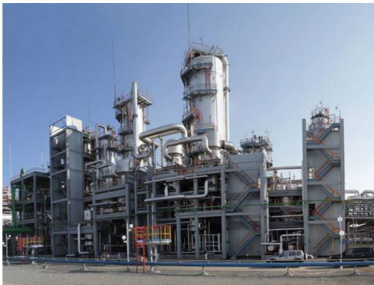
Figure 9.47: Fibrant's oxanone technology of uncatalyst cyclohexane air oxidation process was implemented at Kuibyshev Azot in Togliatti ( https://www.fibrant52.com/en/licenses ).
