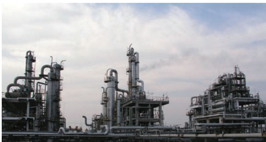
Figure 14.31: The 200 kt/y cyclohexanone oxime industrial production unit. From B. Zong, B. Sun, S. Cheng, X. Mu, K. Yang, J. Z. Zhao, X. Zhang, W. Wu, Green production technology of the monomer of Nylon-6: caprolactam, Engineering, 2017, 3, 379–384. http://dx.doi.org/10.1016/J.ENG.2017.03.003 . Open access.
