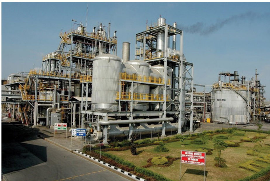
Figure 9.32: Petrowidada phthalic anhydride plant in Gresik, Indonesia.
