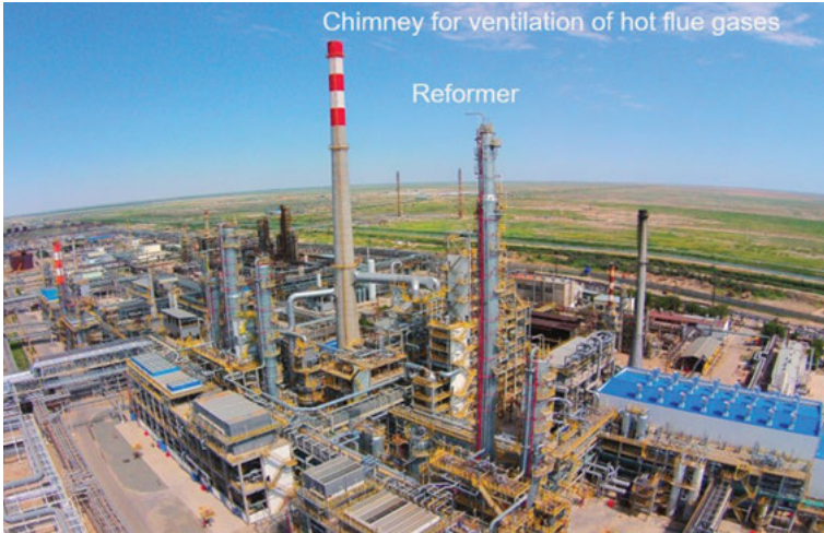
Figure 7.10: Catalytic reformer for processing 1 million tons of the feed annually. The unit at Atyrau refinery in Kazakhstan gives the product with RON of 103.
