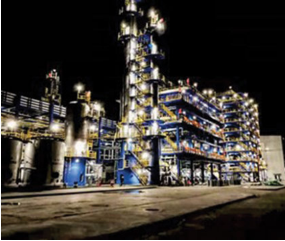
Figure 12.18: PetroChina Harbin Petrochemical Co. Ltd.'s Heilongjiang plant of 150,000 tones per year capacity which uses Ionikylation process. From https://www.hydrocarbonprocessing.com/magazine/2020/april-2020/special-focus-clean-fuels/safe-and-sustainable-alkylation-performance-and-update-on-composite-ionic-liquid-alkylation-technology .
