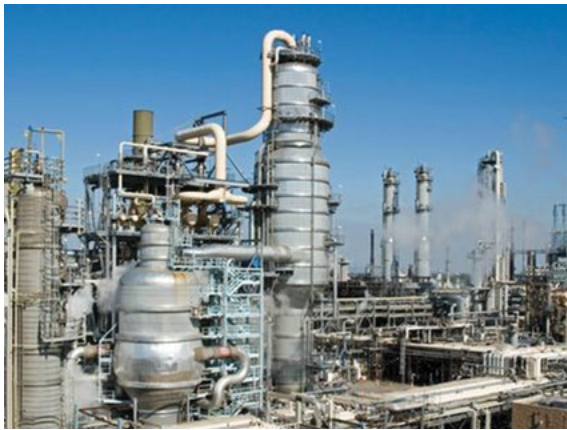
Figure 4.17: Crude oil distillation with a vacuum column on the left and atmospheric crude distillation on the right. From https://www.emerson.com/resource/image/1469794/landscape_ratio4x3/414/310/2abb06010f23415dccc80a6b1990a541/ve/h003-crude-vacuum-unit.jpg .
