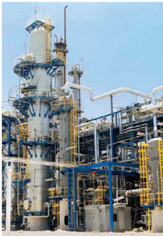
Figure 8.11: Oxychlorination reactor. From https://ucpcdn.thyssenkrupp.com/_legacy/UCPthyssenkruppBAIS/assets.files/products__services/chemical_plants__processes/polymer_plants/uhde_brochures_pdf_en_3.pdf .
