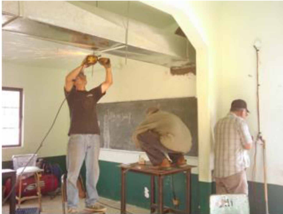
Figure 8. Conditioning of the work center
