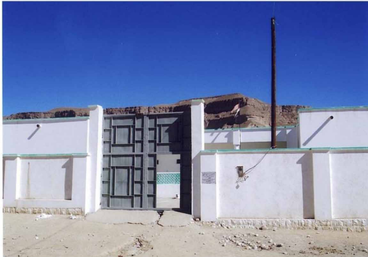
Figure 5. New school, gate and perimeter wall surrounding courtyard, Asnab
