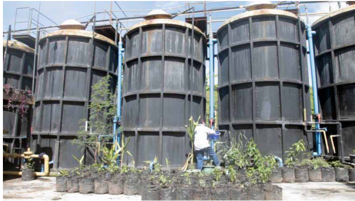
Figure 3. A six-staged fixed-bed anaerobic wastewater treatment plant of tofu wastewater in Sumedang, Indonesia
