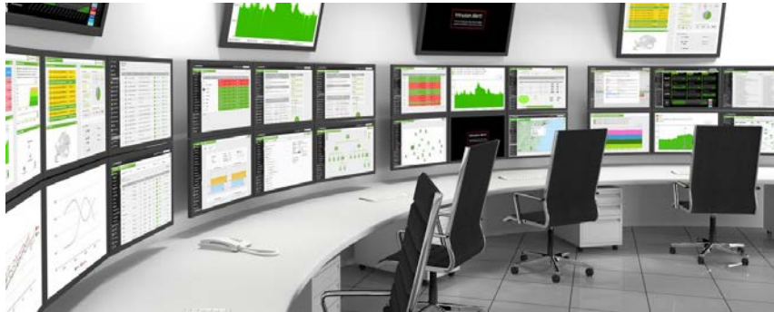
Figure 1.4 – The OTS of the plant is similar to the control room
