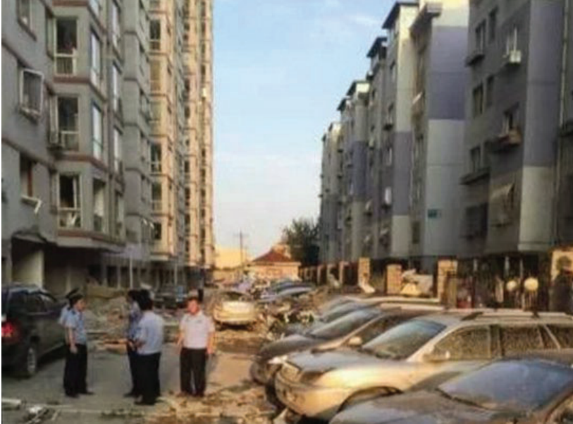
Figure 1-2 A photo from the scene of a gas explosion in a Dalian district
