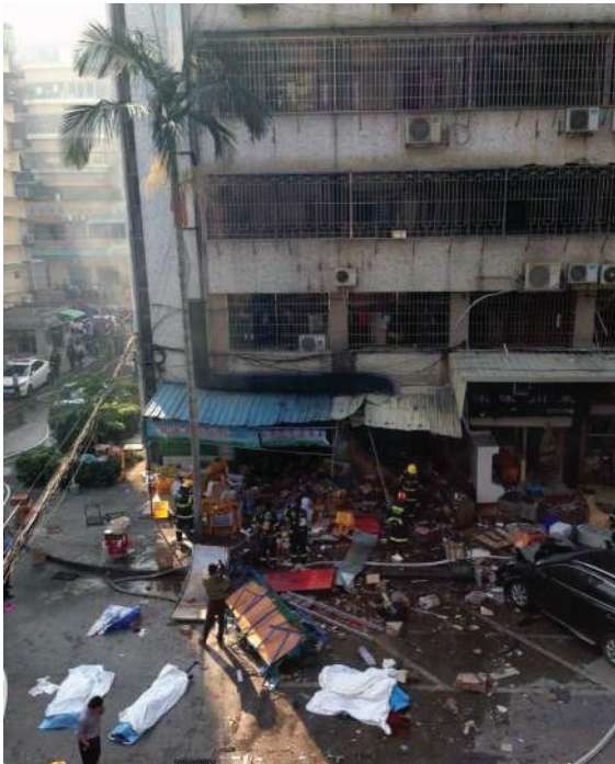
Figure 1-7 Scene of the accident at Xiamen gas explosion
