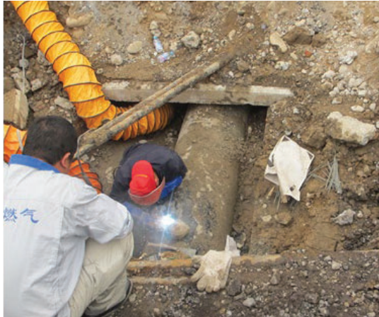
Figure 1-4 Photograph of the gas line rehabilitation process
