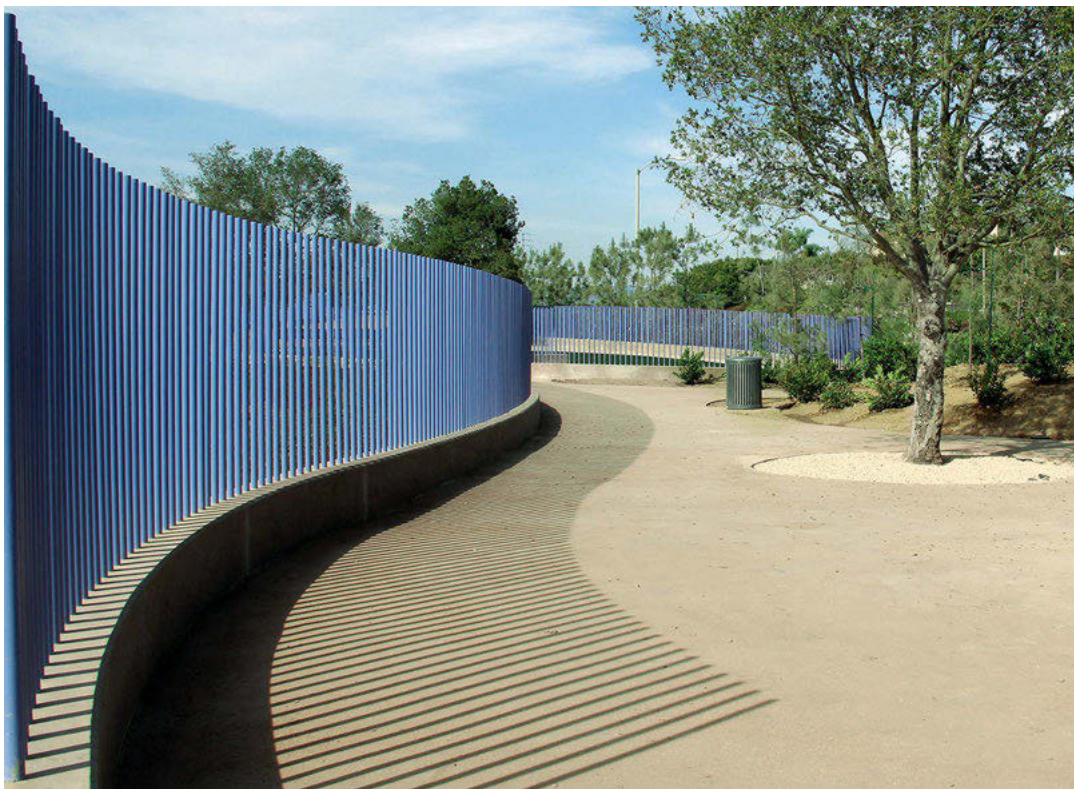
Powder-coated steel poles embedded in a cast concrete base form an elegant and relatively economical fence at the Newport Beach Civic Center and Park , California, 2013. [Photographed 5 years after construction]
