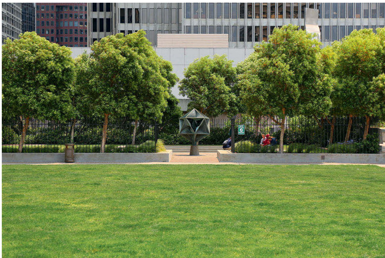
Alcoa Plaza in San Francisco, 1961, presents a highly legible example of an on-structure landscape where soil beds sit above the supportive podium and vary in thickness according to planting needs. [Photographed 57 years after construction]
