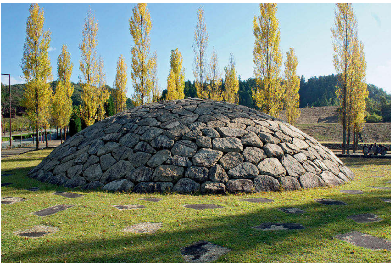
Stone boulders are interlocked without mortar to create an iconic element at Harima Science Garden City , 1994. [Photographed 18 years after construction]
