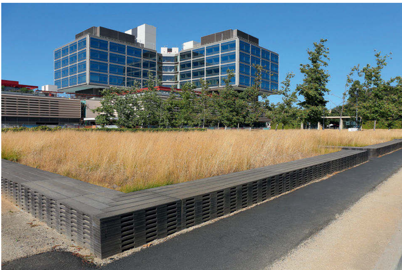
Medical Center Parking Structure 4 , Stanford University, 2003. With the parking garage embedded below ground, this thin and relatively lightweight rooftop garden has the feeling of simply being a continuation of the surrounding landscape. [Photographed 15 years after construction]
