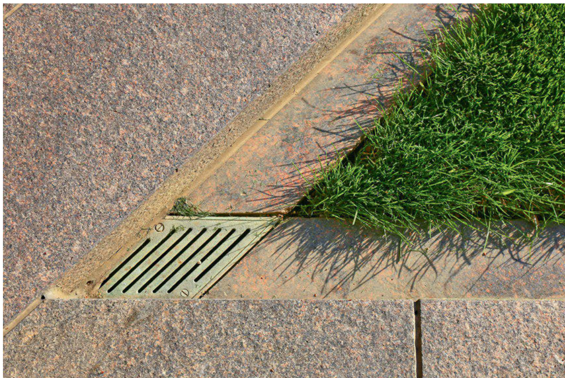
Detailing of paving edge allows for shadow between walkway and adjacent turf, emphasizing flatness at Burnett Park , Fort Worth, 1983. [Photographed 35 years after construction]
