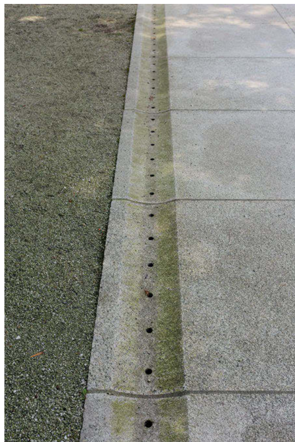
Monolithic stone paving with integrated drainage channel at its perimeter within The Forum at Novartis Campus , Basel, 2007. [Photographed 11 years after construction]
