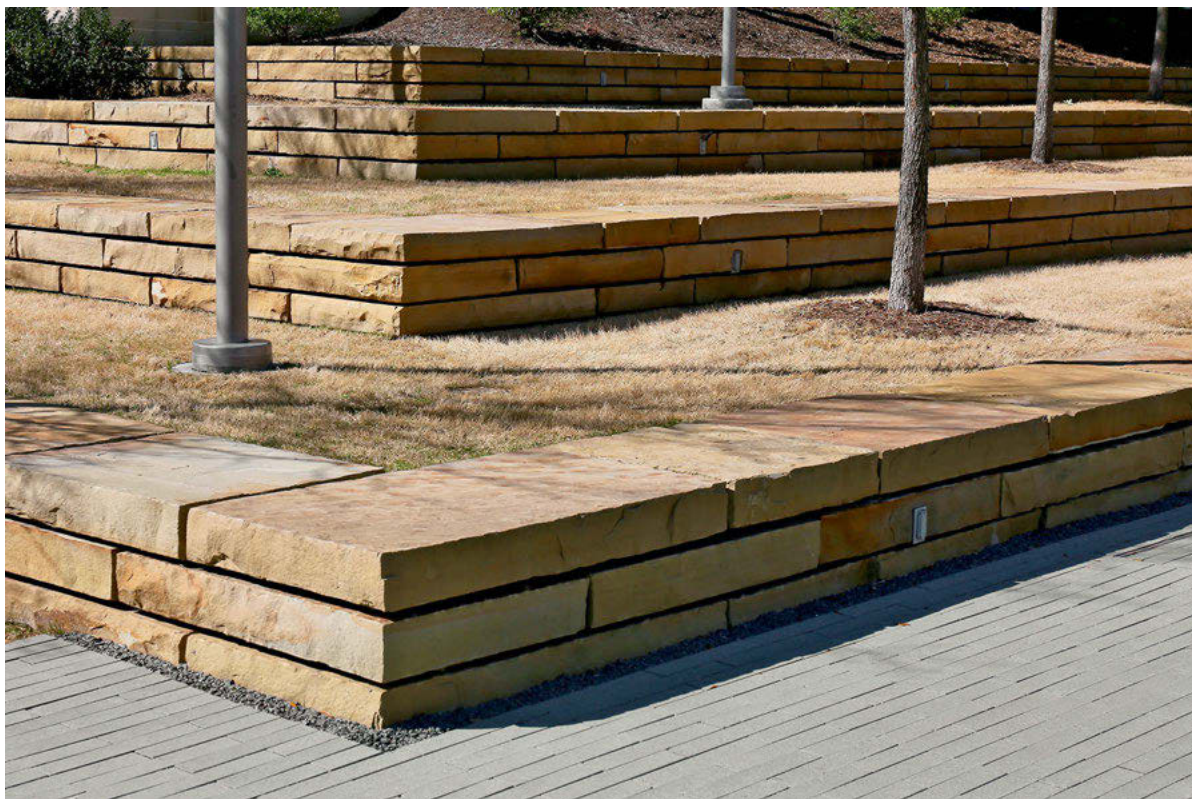
Stone seatwalls and colored precast concrete pavers enhancing the campus of University of Texas at Dallas, 2011. [Photographed 7 years after construction]
