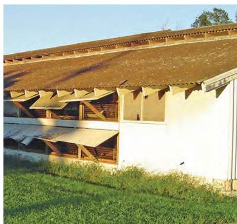
Fig. 21.5. A rabbitry in Louisiana constructed with roof vents to aid air movement by the “chimney effect.” (Courtesy of J.I. McNitt)
