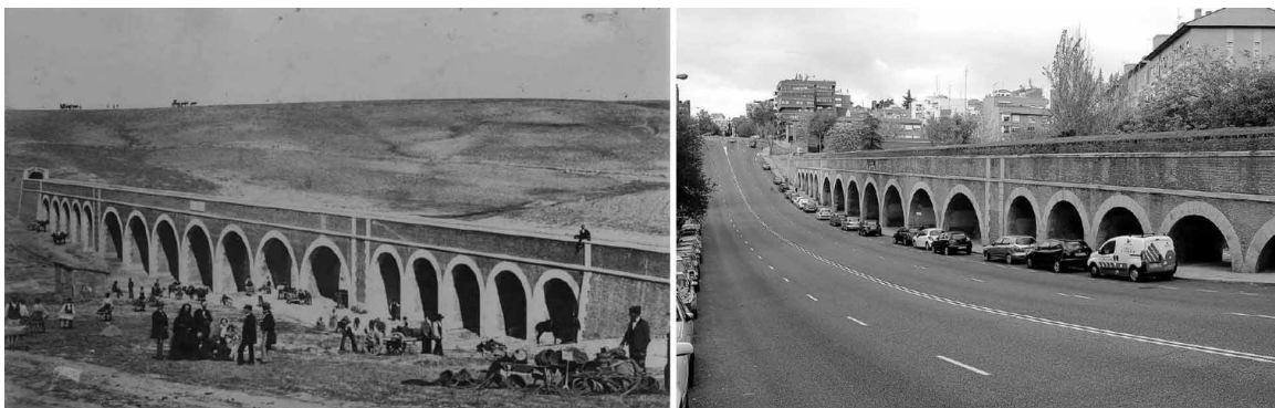
Figure 6. Construction of the Amanuel Canal or Viaduct. Source: Charles Clifford’s Archive (1856) Amanuel Canal or Viaduct today along the Pablo Iglesias de Madrid Street. Source: author’s picture (2013)
