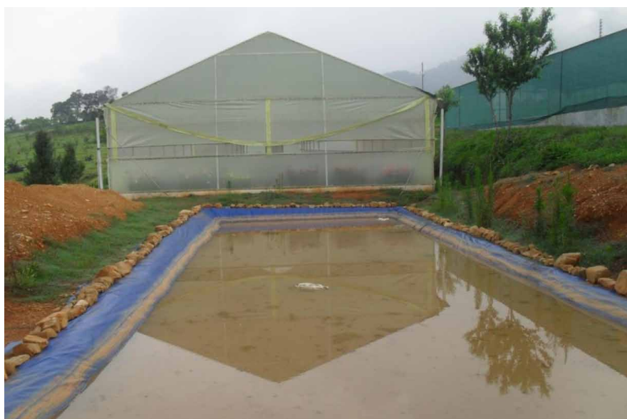
Figure 21. Rainwater harvesting technology
