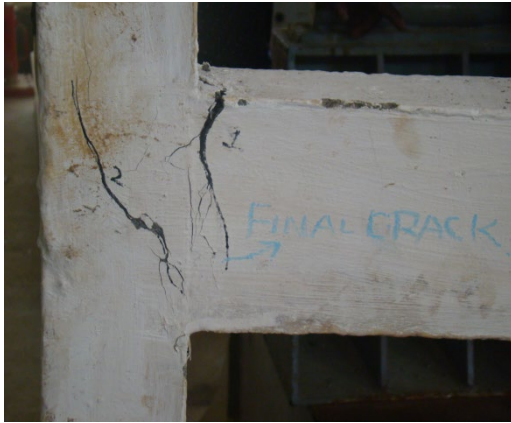
Fig. 3. Cracks in CM Specimen
