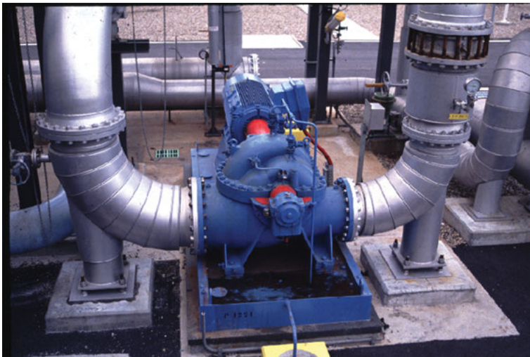
Figure 16.1: Typical heavy-duty horizontal end-suction process pump.
