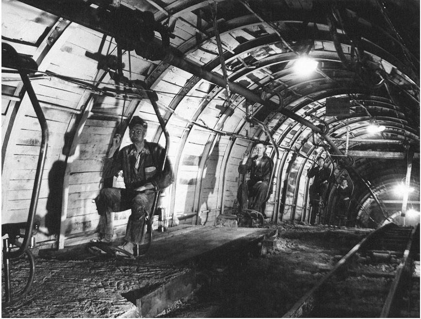
Figure 4.14 The Hunt Rider cable cars at Babbington (photo credit: Coal Authority)
