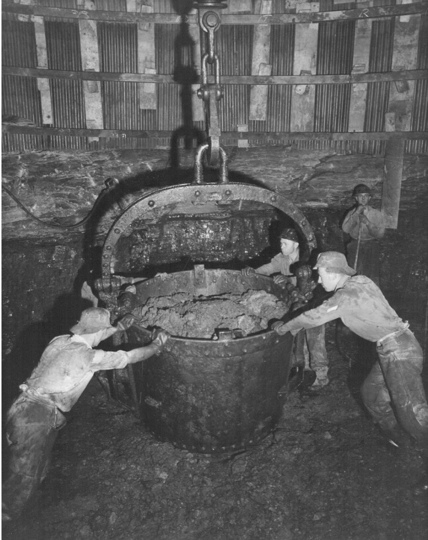
Figure 4.8 Shaft sinking at Bevercotes Colliery in the late 1950s (photo credit: Coal Authority)
