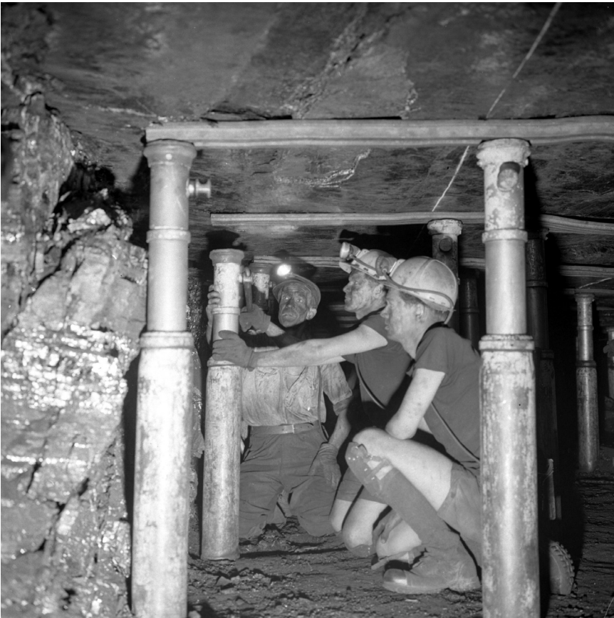
Figure 4.10 Props (photo credit: Coal Authority)
