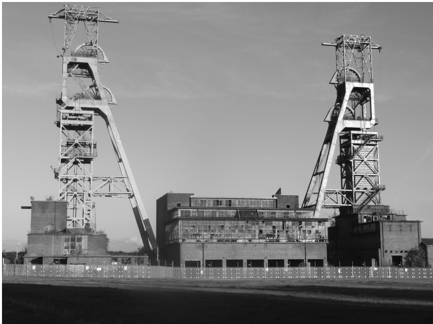
Figure 4.18 Headstocks and winding gear at Clipstone
