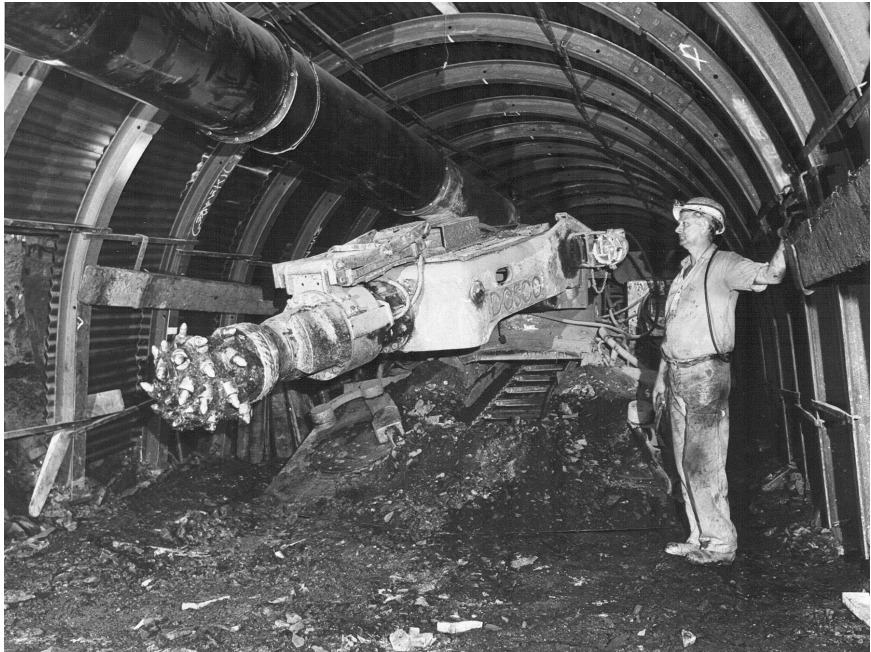
Figure 4.12 DOSCO roadheader (photo credit: Coal Authority)
