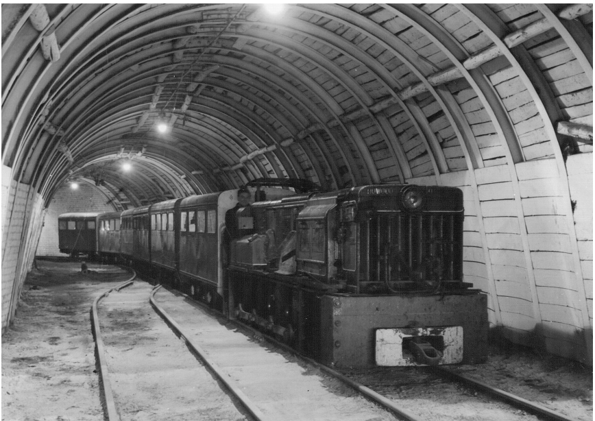
Figure 4.15 Underground manriding train at Thoresby (photo credit: Coal Authority)
