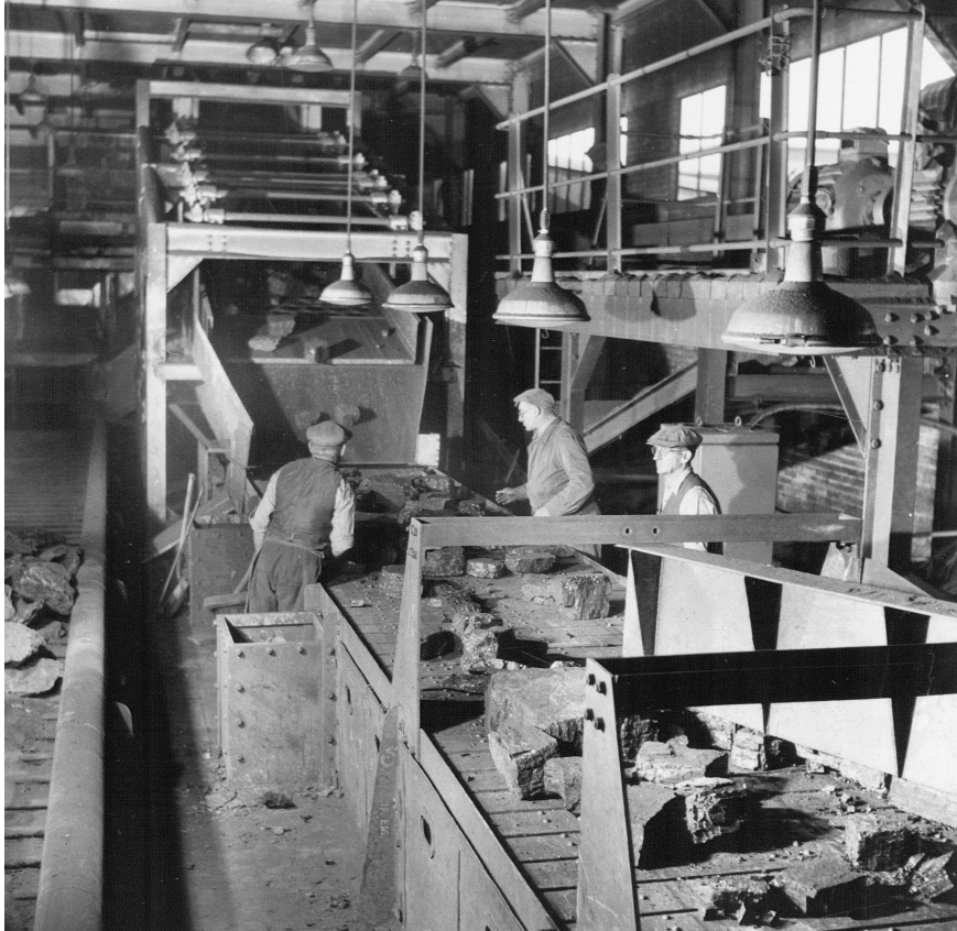
Figure 4.19 Coal preparation plant at Mansfield Colliery (photo credit: Coal Authority)
