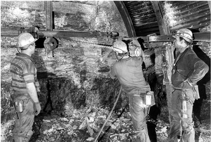
Figure 4.3 Drilling at Shirebrook Colliery in the late 1970s (photo credit: Mansfield and Ashfield Chad)
