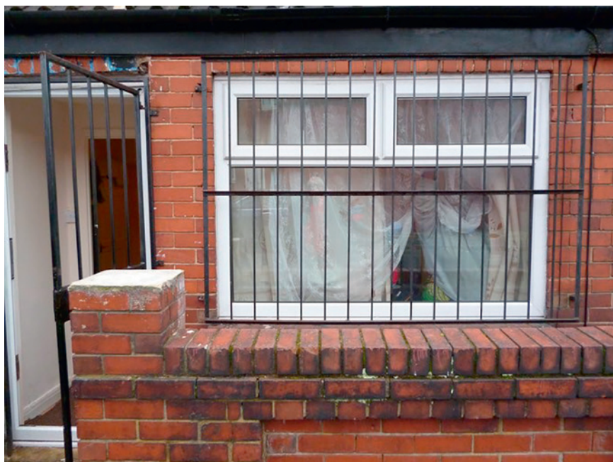
Figure 5.3 Bars covering front windows of house used for asylum seeker accommodation.
