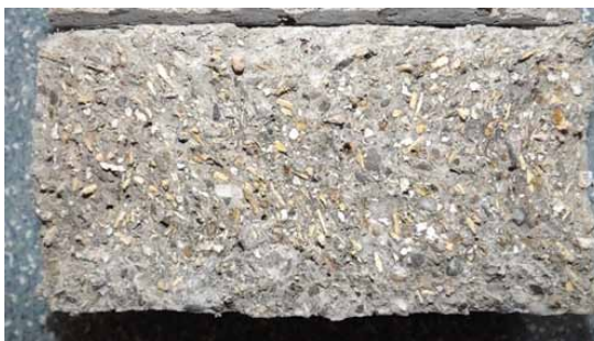
Figure 2. Transversal section appearance of the concrete with SSA
