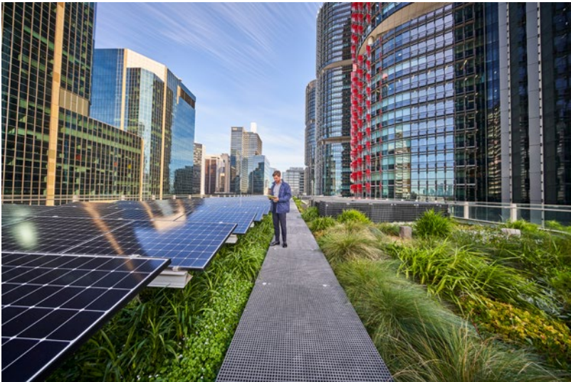
Daramu House green roof and solar panels. Source: Lendlease
