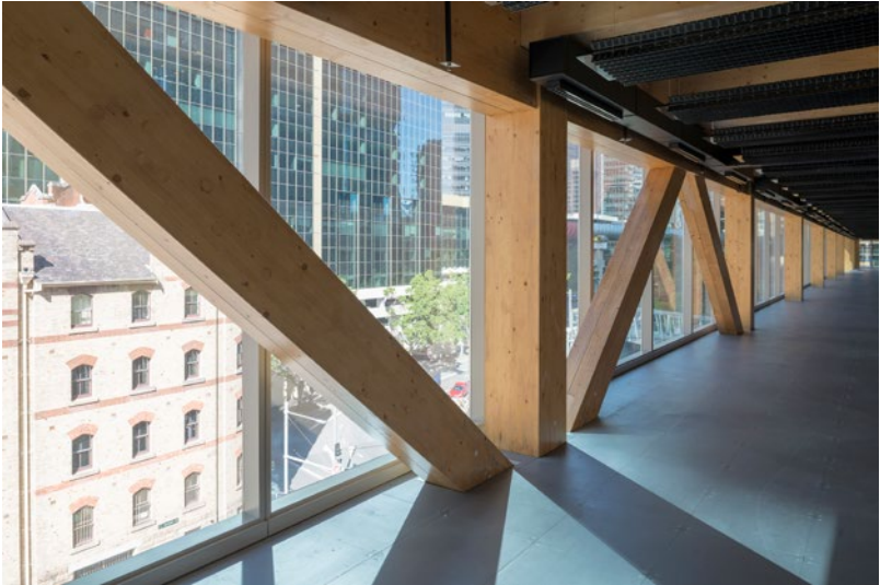
Lendlease constructed Daramu House from engineered timber. Source: Lendlease
