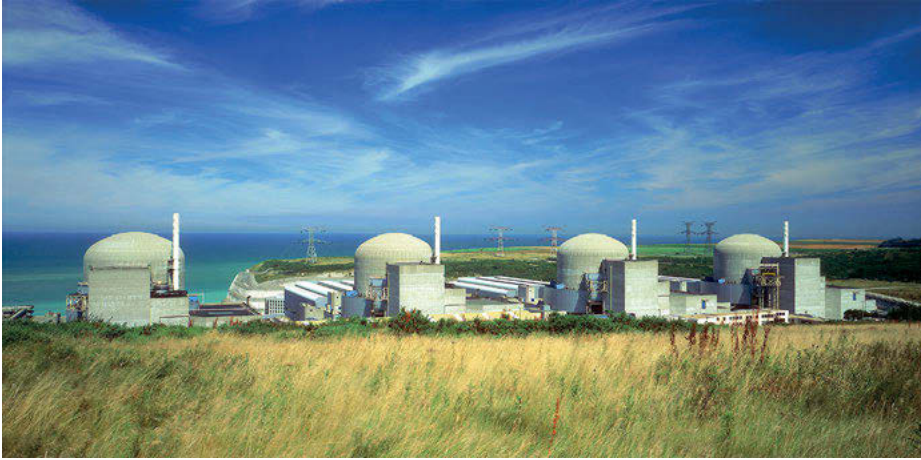
Fig. 10.9: Paluel Nuclear Power Plant with four 1300 MW eI PWR units in Normandy (Northern France) (© AREVA, Laurence Godart).
