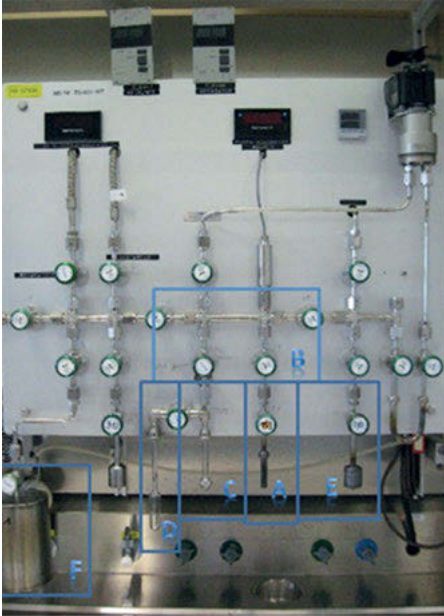
Fig. 11.15: TRITEC AG (Switzerland) uranium trap system allowing safe handling of tritium gas. Careful heating of the storage vessel (A) containing depleted uranium releases tritium gas ( T_2 ) into the compartment (B). Controlled release into the reaction compartment (C) allows exact determination of the added amount of tritium gas. From the pressure difference (before and after release into the reaction compartment), the volume of compartment B and the specific activity of the tritium gas the exact amount of activity (tritium gas) released to compartment C can be calculated. After completed reaction, there is reabsorption of the unreacted amount of tritium gas to the waste vessel (E). As a safety measure, an additional vessel (F) allows the complete retention of the volatile activity avoiding any release to the environment.
